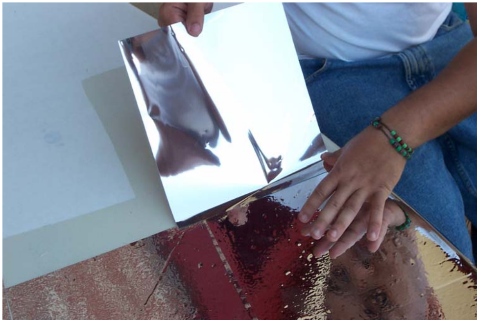
Figure 2.2: Application of Aluminized Mylar to Fiberglass Panels of the Dish
