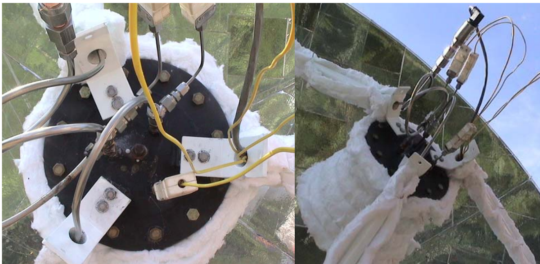
Figure N.11: Receiver/boiler assembled at the focal region of concentrator.
