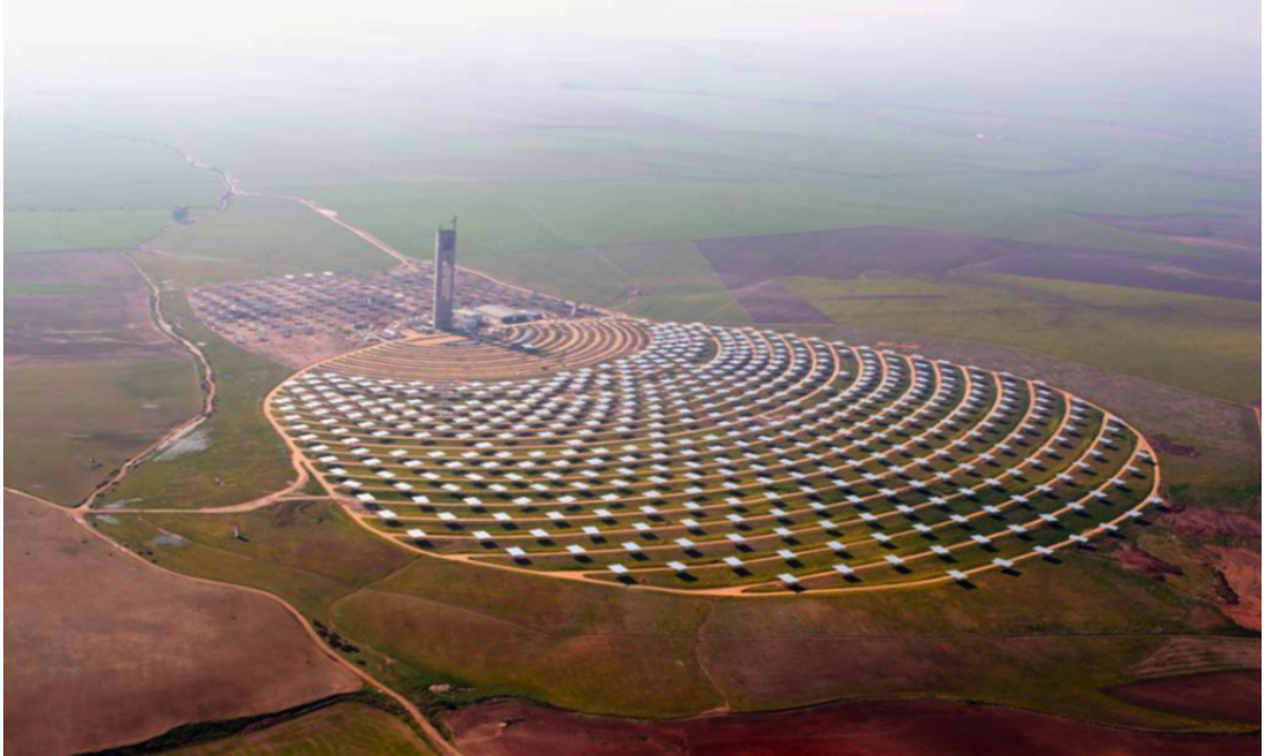
FIGURE 2.2. PS-10 in Seville Spain, built by Abengoa Solar, has an 11MW installed capacity and is the first commercial solar power tower in the world.
