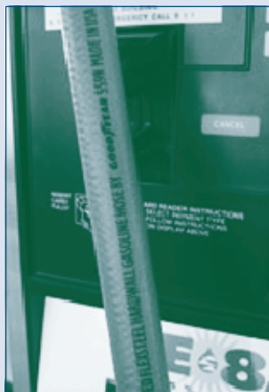
Always use an E85-compatible hose on E85 dispensers.
