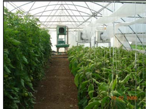
Figure 15: PE chimneys in ATES greenhouse
