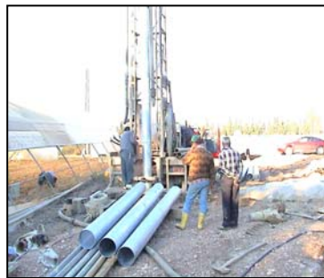
Figure 6: Casing and gravel pack
