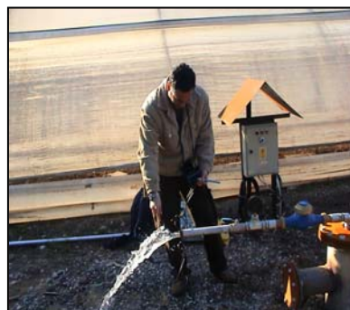
Figure 7: Long term pump test
