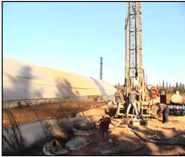
Figure 2: Well drilling
